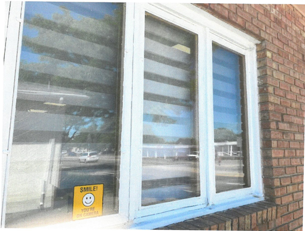
North side window (cracked, rotting)
